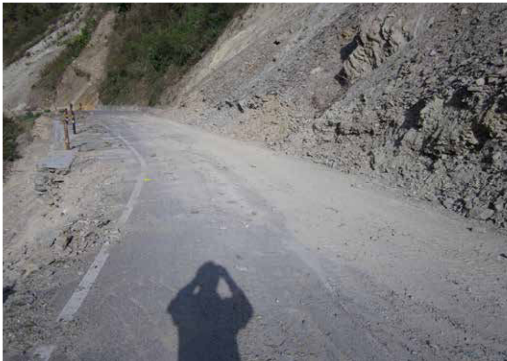
Picture 8: Breast wall constructed along the chainage 3 + 000Km on Hanumanti-Fatehpur road
