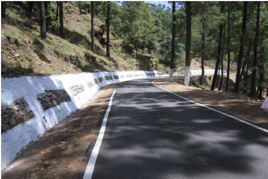
Picture 7 Breast wall constructed along the chainage 3 + 000Km on Chailusain-Devikhet road
