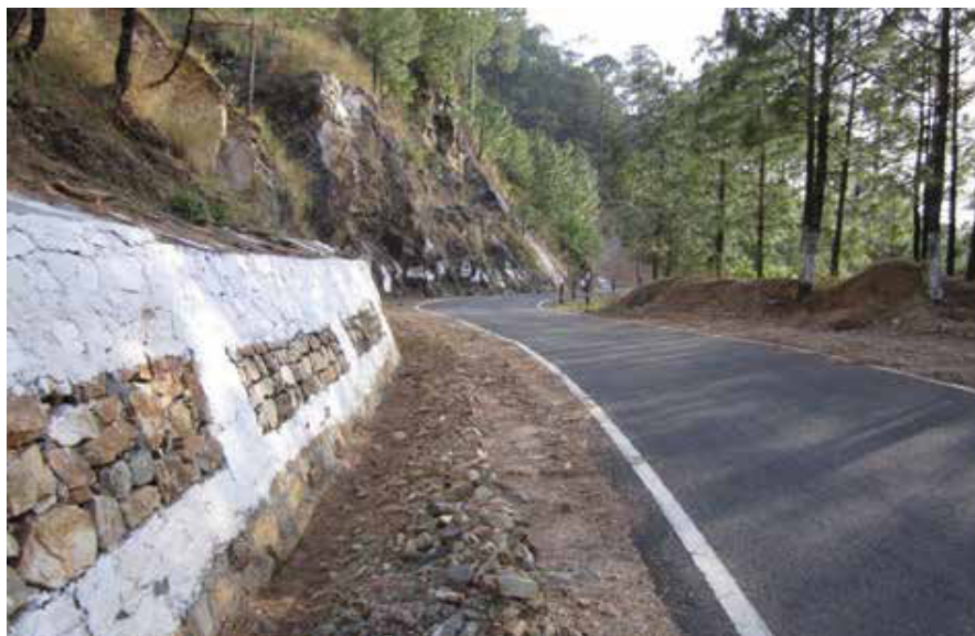
Picture 2 Breast wall constructed along the chainage 6 + 730 Km on Kandakhal-Chailusain road
