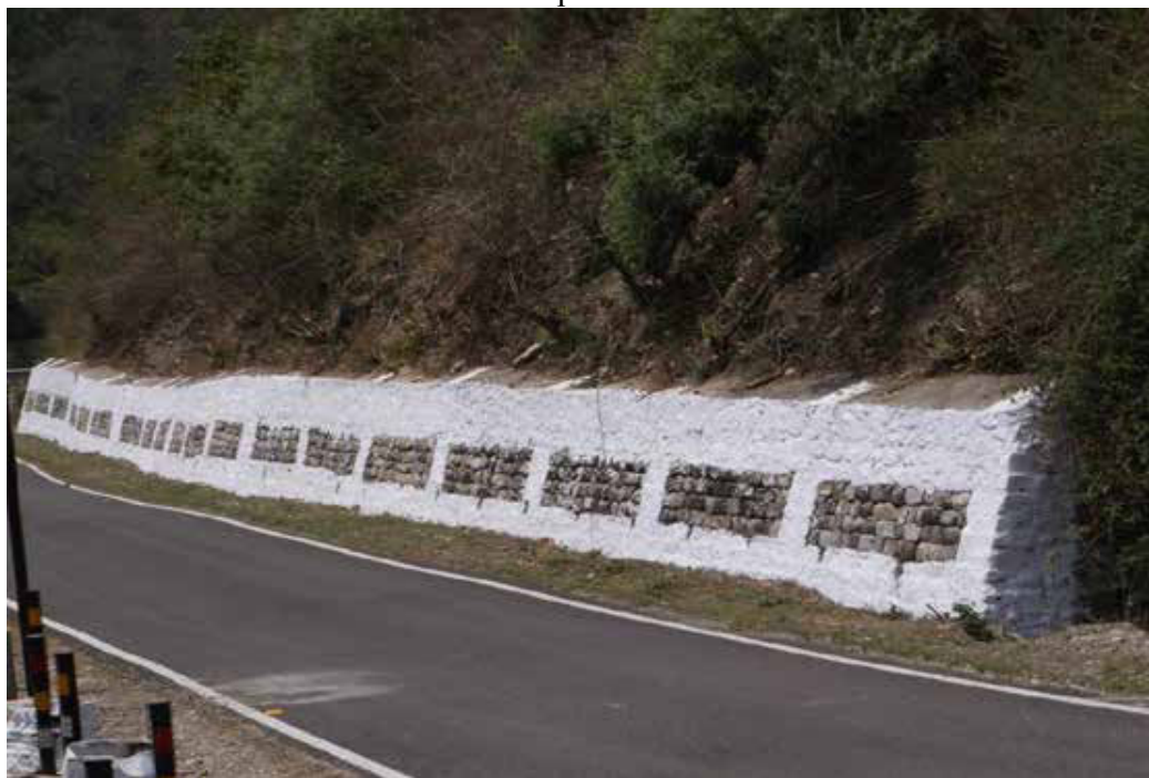
Picture 10: Breast wall constructed along the chainage 13 + 400Km on Hanumanti-Fatehpur road
