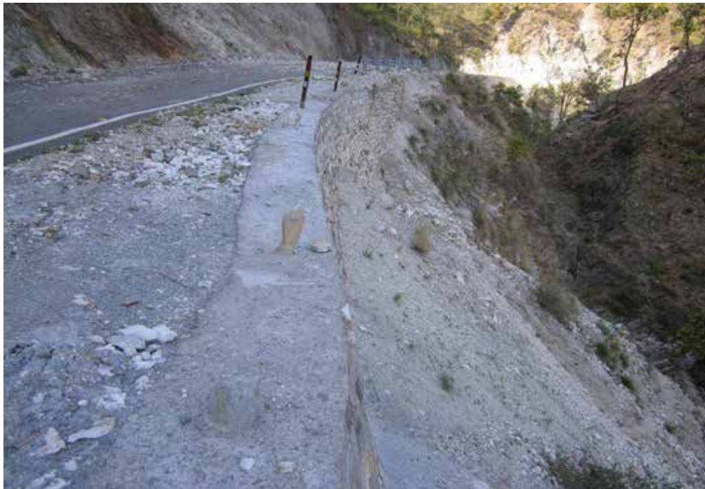
Picture 9: Retaining wall constructed along the chainage 3 + 000Km on Hanumanti-Fatehpur road
