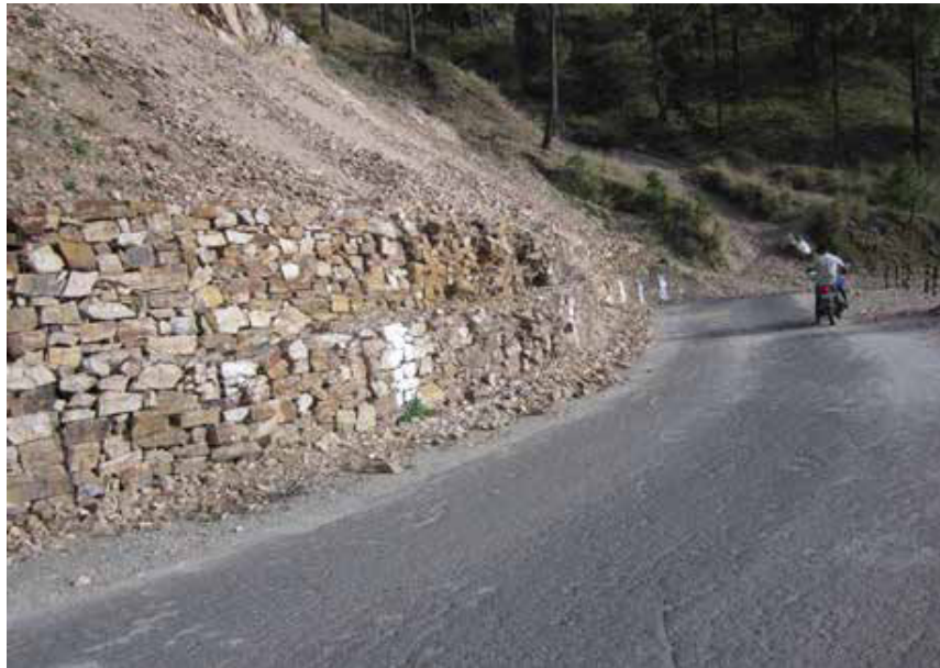
Picture 1: Wire-Crete under construction along the chainage 10 + 650Km on Kandakhal-Chailusain road
