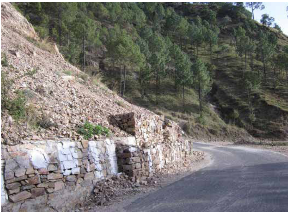
Picture 4 Wire-Crete constructed along the chainage 8+400 Km on Matiyali-Dwarikhal road.
