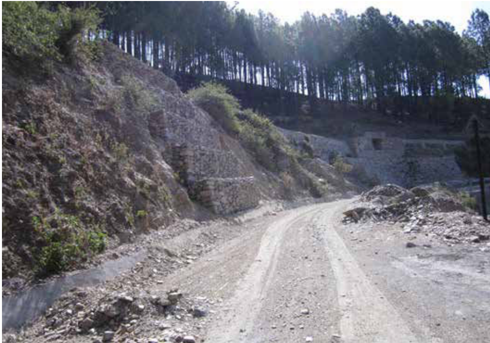
Picture 3 Wire-Crete constructed along the chainage 14 + 600Km on Matiyali-Dwarikhal road
