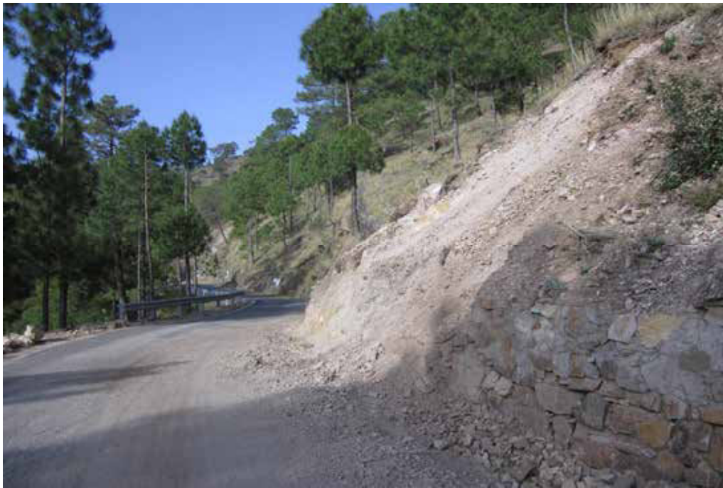
Picture 5 Breast wall constructed along the chainage 6 + 900Km on Matiyali-Dwarikhal road.
